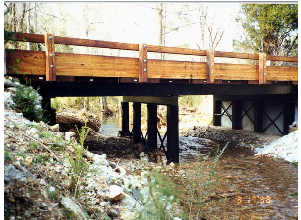
Vehicular Timber Bridge, Floyd County
